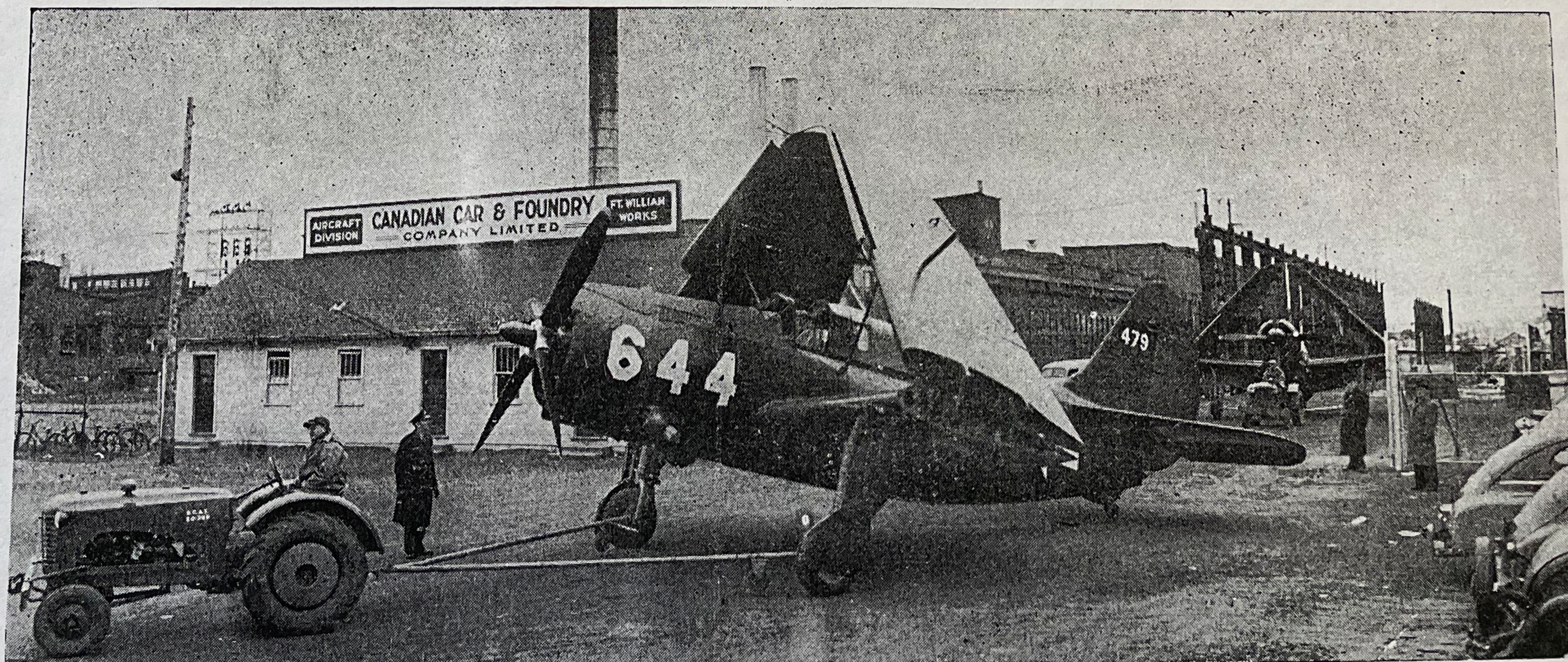
Completely tested both for engine performance and armament, this Helldiver leaves the plant for the airport where she will take to the air on her initial flight.
